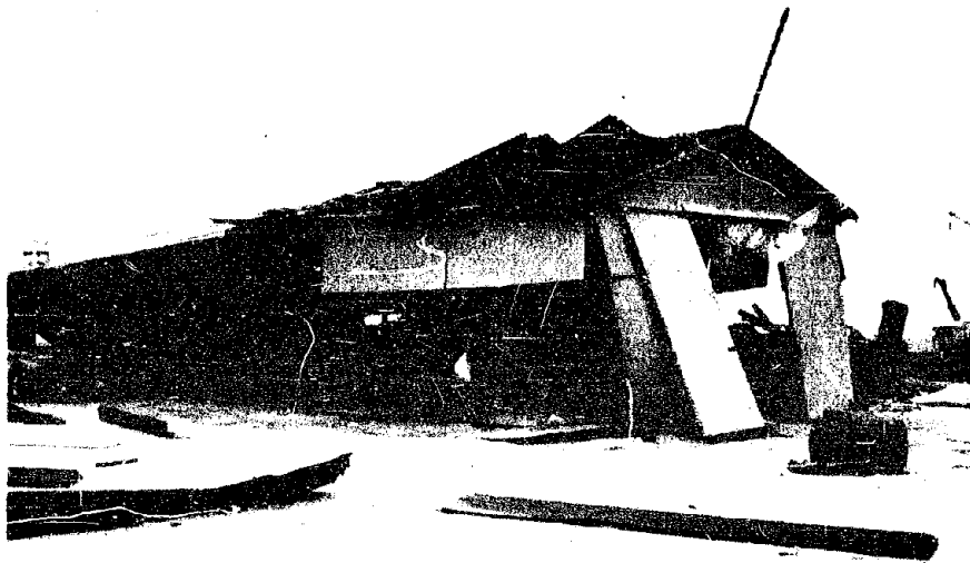
Fig. 3.25 Bin Storage Warehouse Looking Northwest, Tare Island, Postshot, 14-3/4 Miles from GZ
